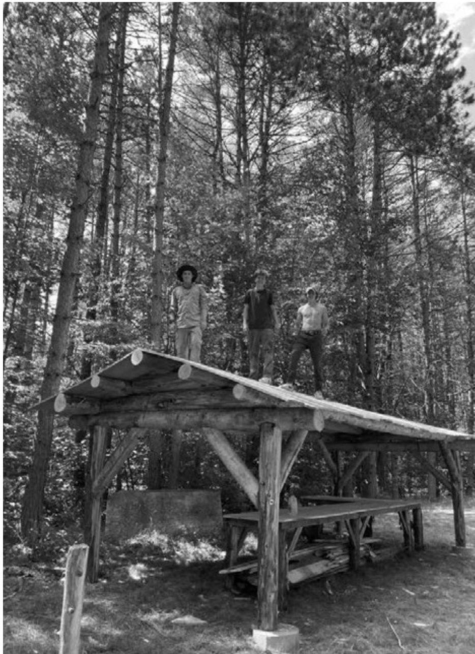
LTIPs at work on the Kababa Pavilion.
