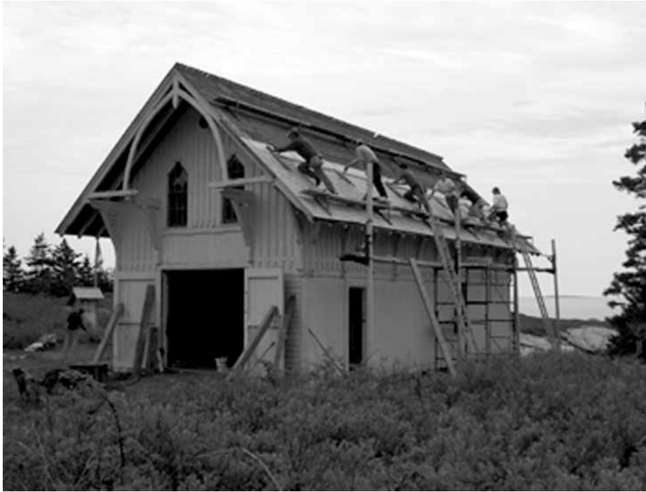
Large crew on the roof
