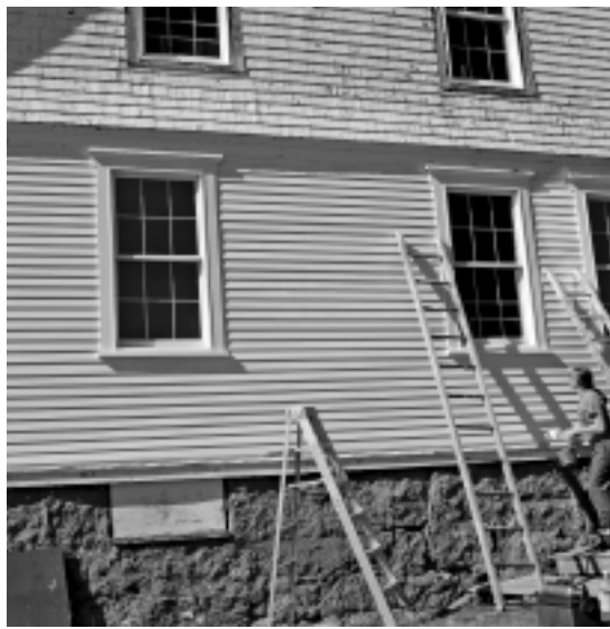
New clapboards on the Keeper's House
