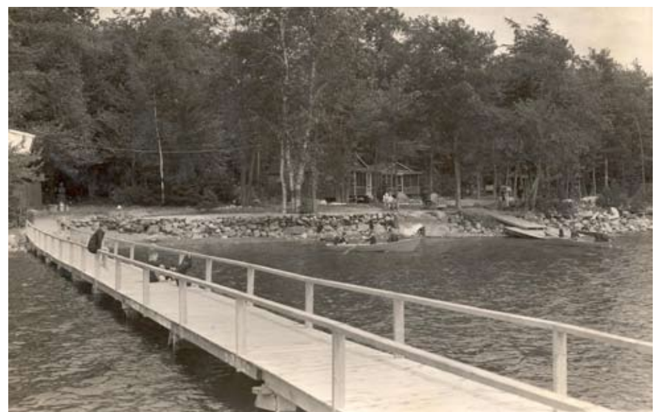
A mainland dock of exceptional length was built to accommodate the low water level in 1941.
