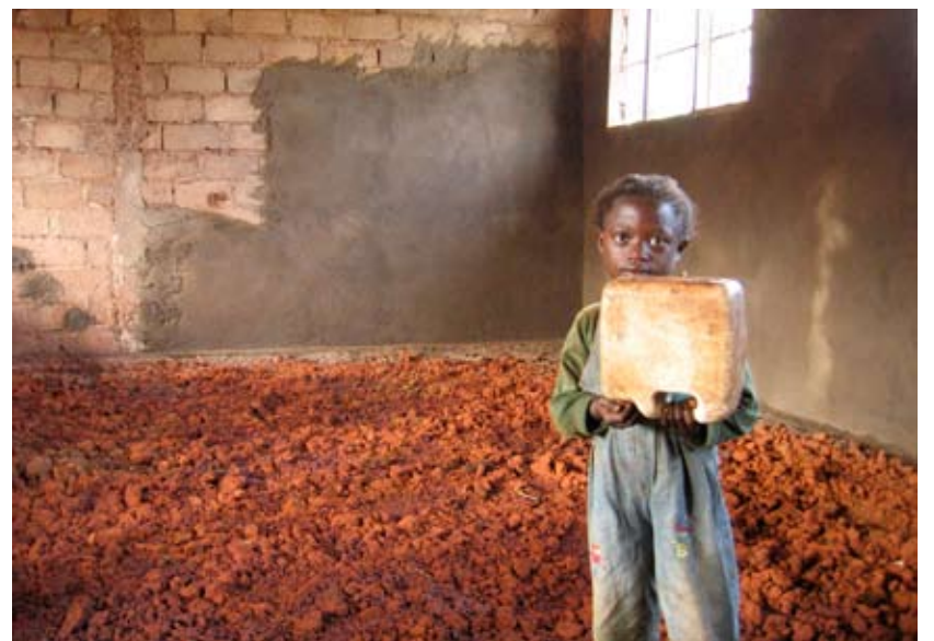
Student helps with classroom restoration. Note partially finished walls.
