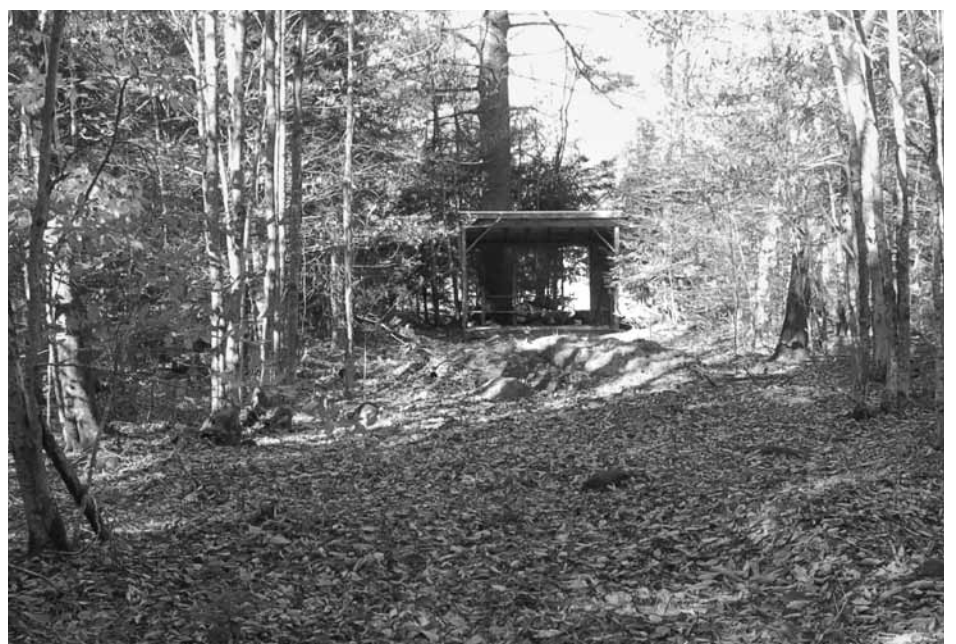
Looking back toward the former riflery firing platform from the end of the new archery range.
