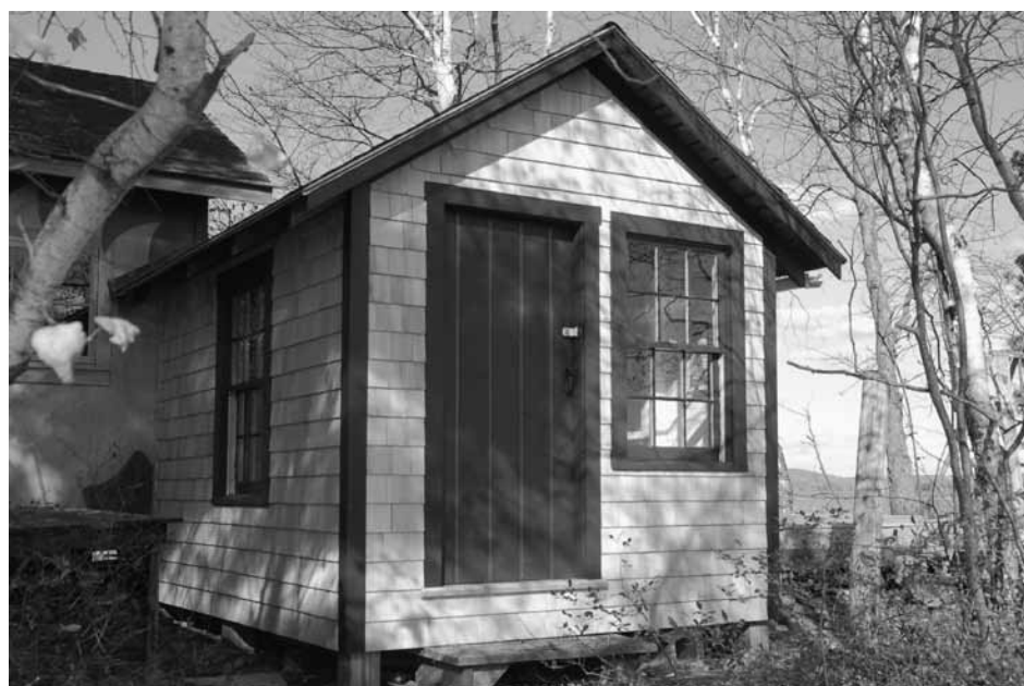
"The Condo" completely refurbished.
