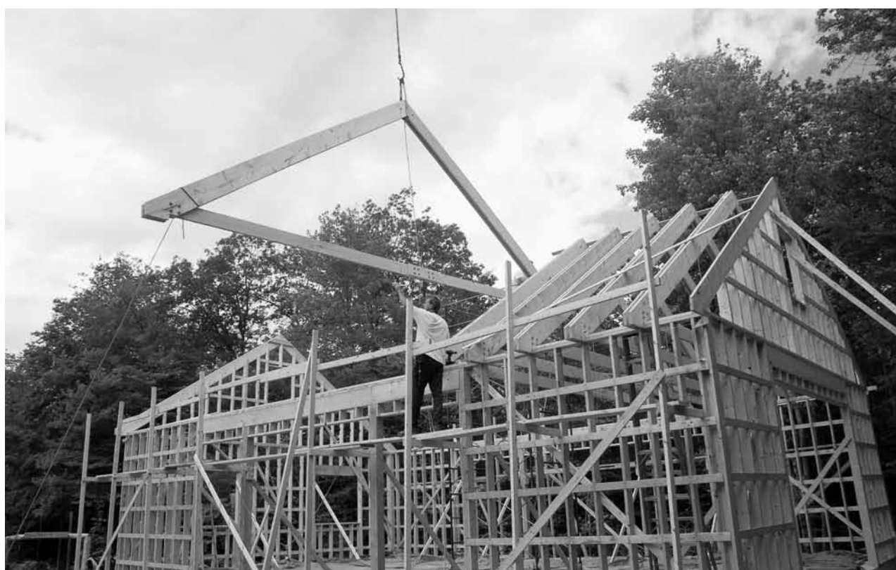
Trusses being lowered into place in May 2013.
