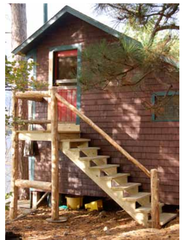
New steps on the South Perch
