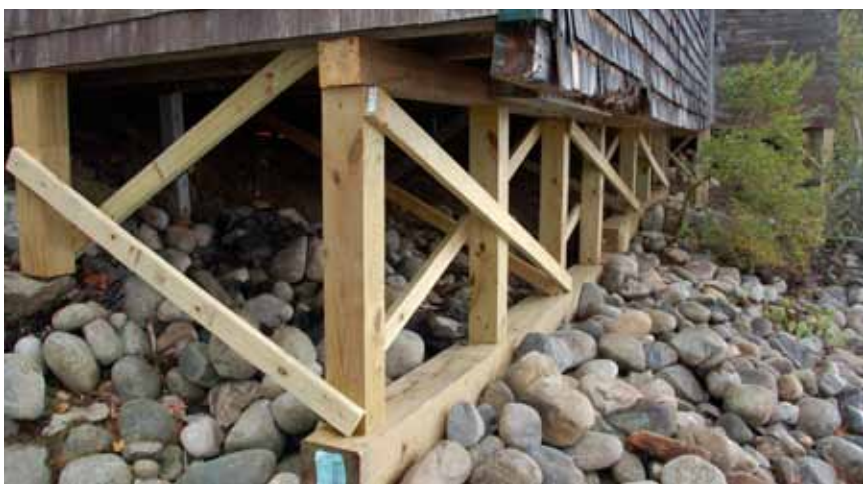
New underpinnings for the O.A.R. Office
