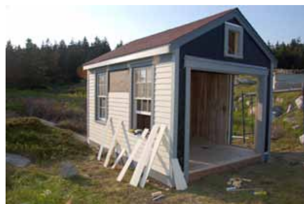
The tractor shed to staff quarters project nearing completion
