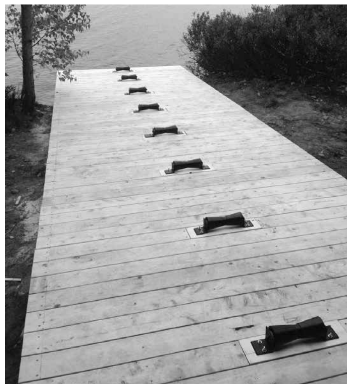
The finished product with built-in disappearing rollers
