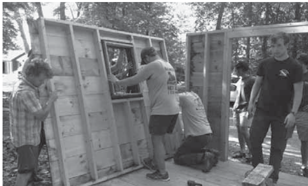
Down come the walls
