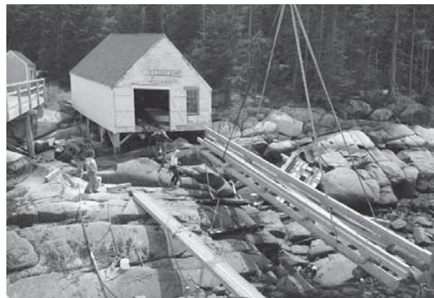
Ramp swinging into place at the Coast Guard boathouse
