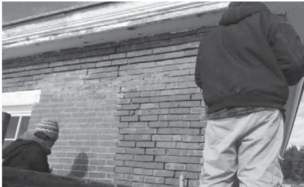
Crew at work repairing and repointing the south wall
