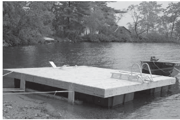
The new swim float ready to receive the diving board
