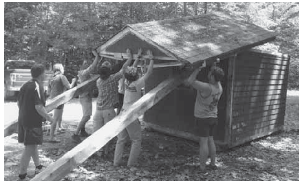
WFR crew taking the roof off the Baita House
