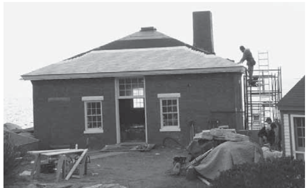
New shingles going on
