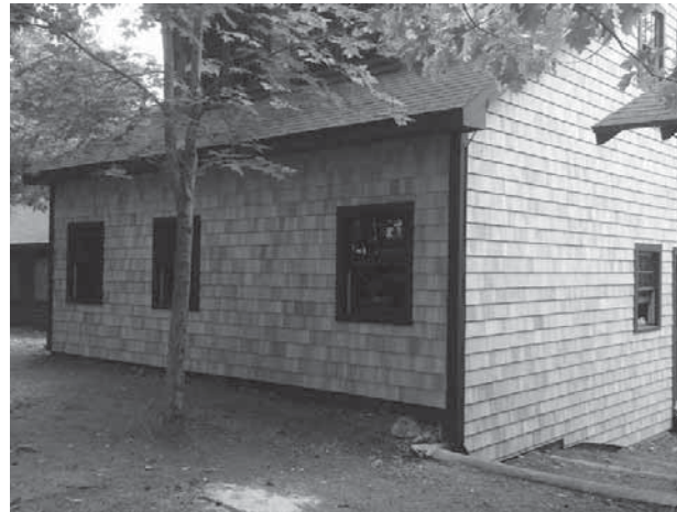
New shingles and trim on the kitchen building
