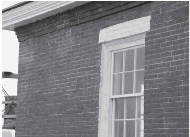
East Wall and soffit repaired!
