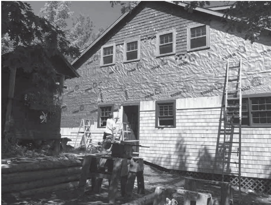
At work on the south wall
