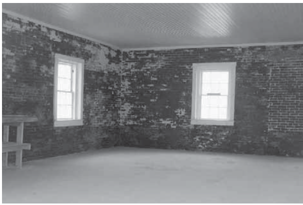
The new floor and ceiling!
