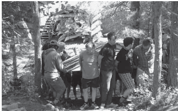
The roof headed up the hill...
