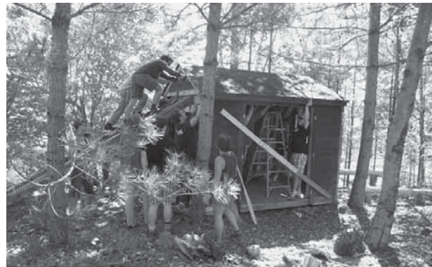
... and back on the building!
