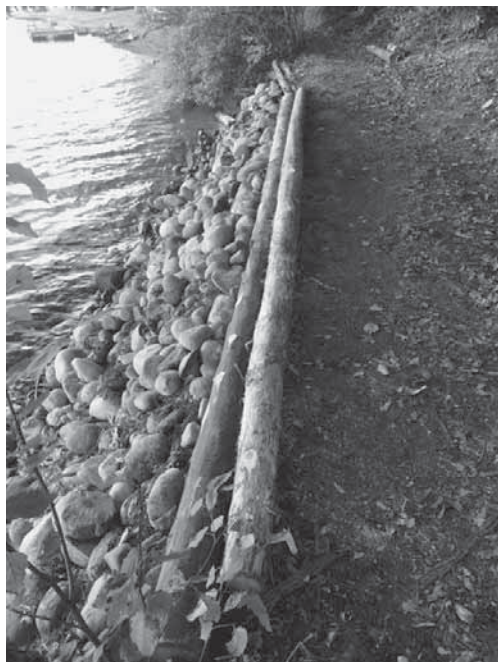
Rebuilt embankment by the dory docks
