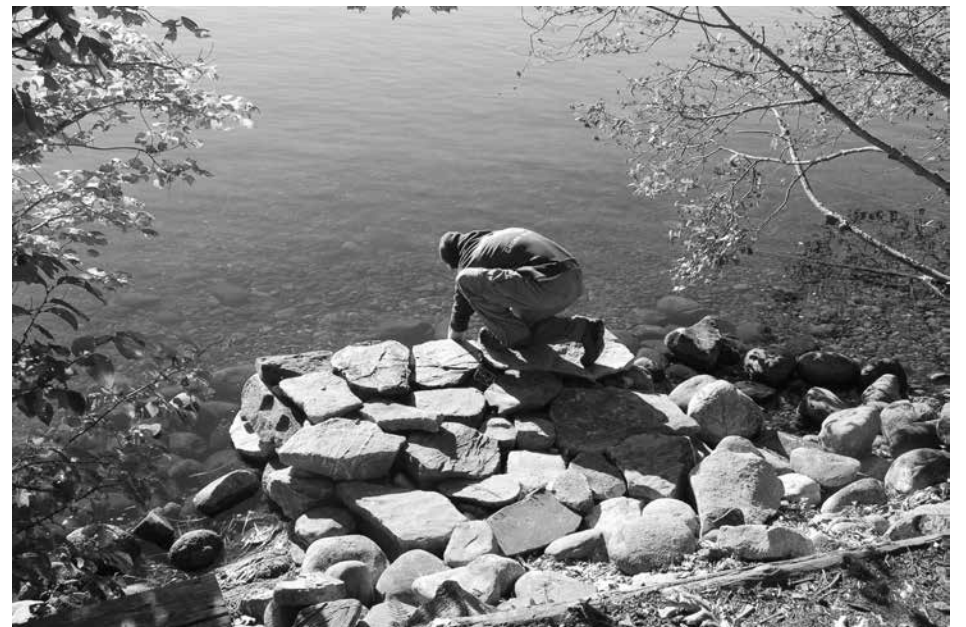
The LTIPs' new hand-washing jetty
