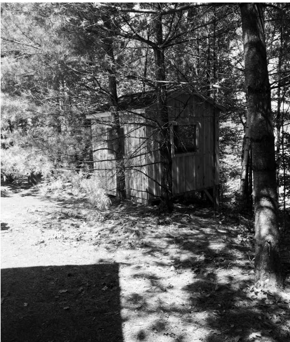
The completed Hermitage nestled in the trees to the east of Honk Hall
