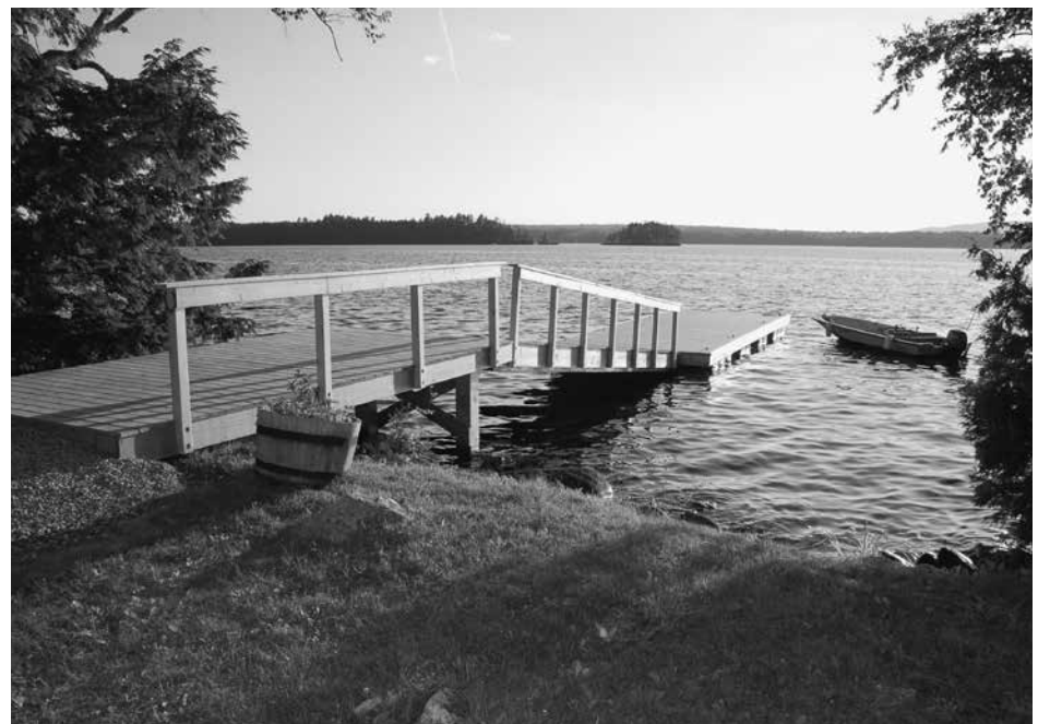
The new Mainland Dock
