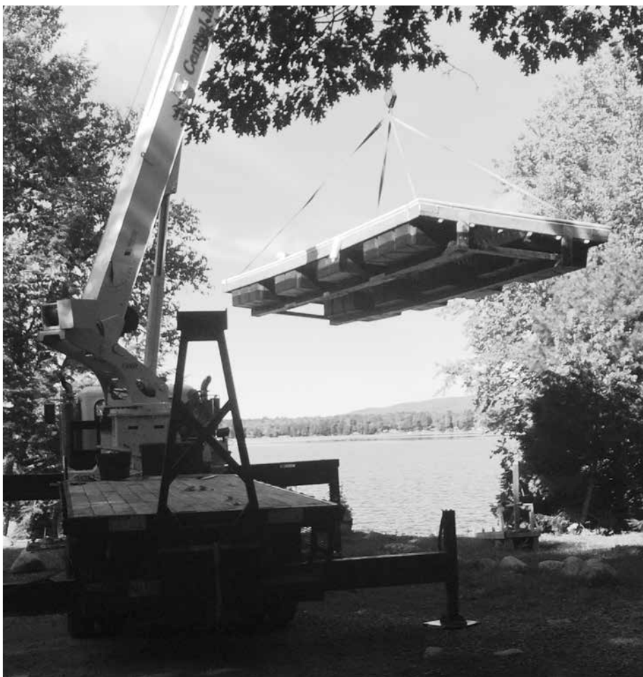
Central Maine Crane moving the float to Great Pond
