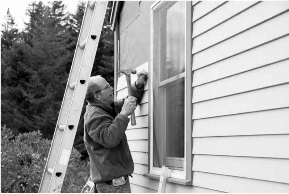
Volunteer James Eklund at work on the new staff house
