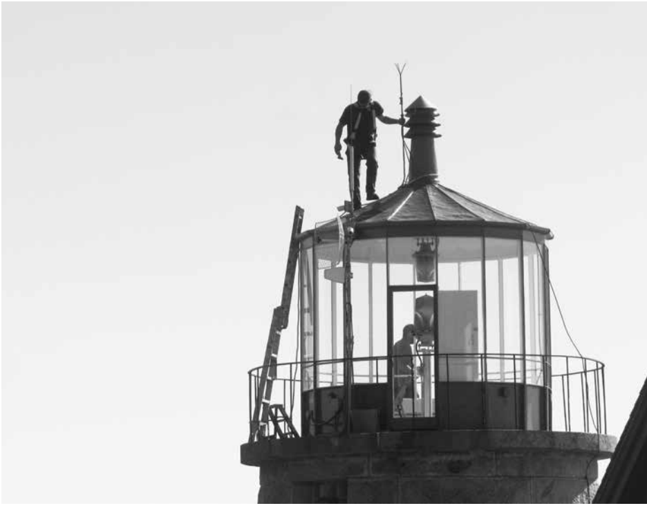
Jim Leslie's crew atop the Whitehead Lighthouse
