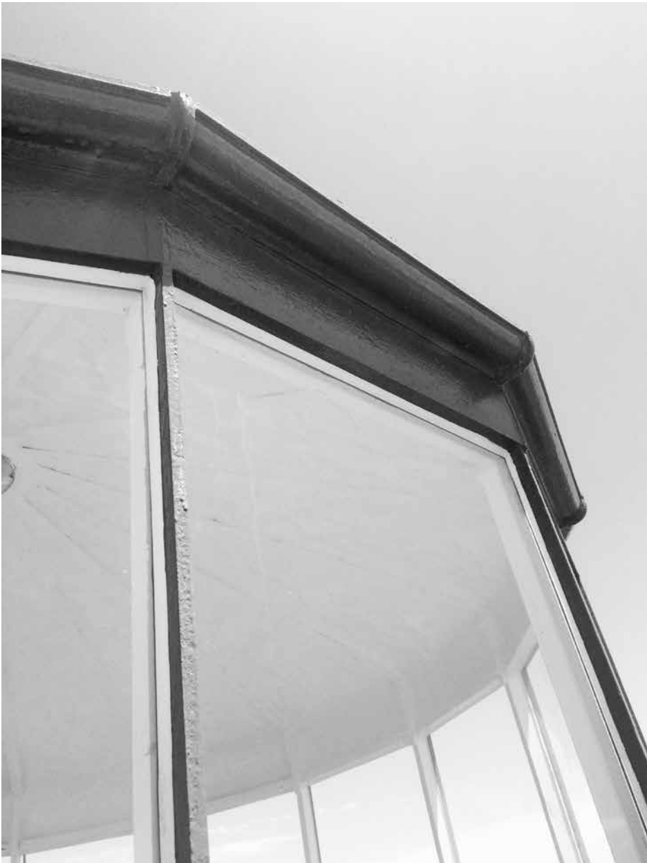
Repaired and painted metal and new glass in the lighthouse
