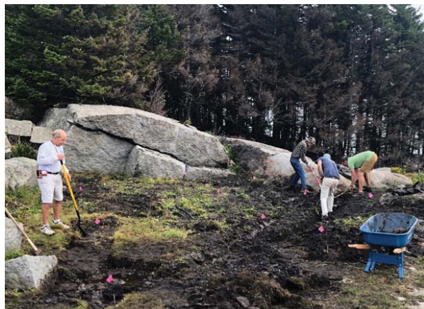
Volunteers preparing the site for the new shop building
