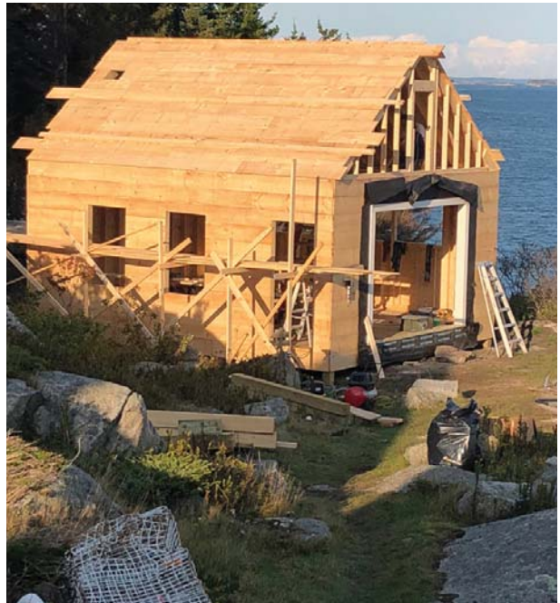
Nearly fully sheathed after just two days' work
