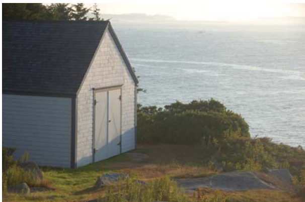
The septic house at Whitehead Light Station before it burned
