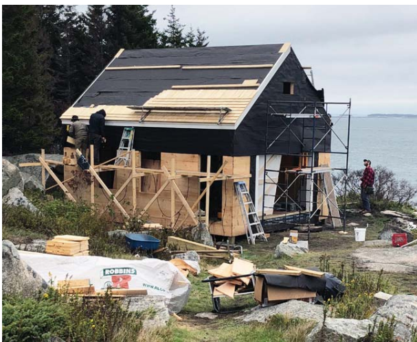
Roof shingles are going on
