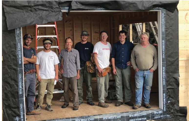
Contractors and volunteers at the end of a day's work on the new shop at Whitehead Light Station: Ben Schachner, Ian Ford, Rob Chandler, Satchel Toole, John Alsop, Charlie Krause, and Nick Buck
