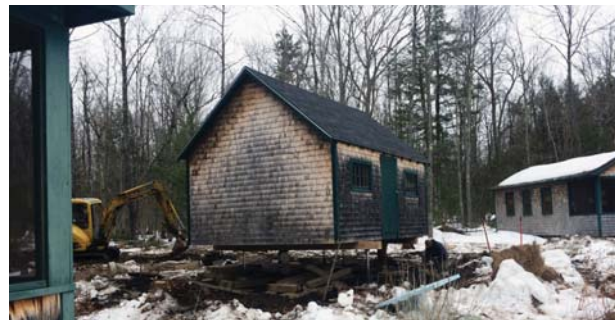
The Santa Maria being lowered into place last winter
