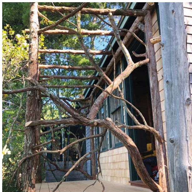
Adirondack-style railings and lattice on the new porch of the Bunkhouse
