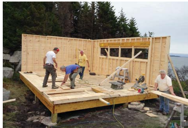
Two walls up and two to go
