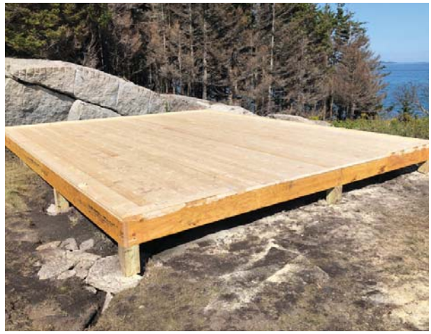
Deck completed awaiting the volunteer framing crew
