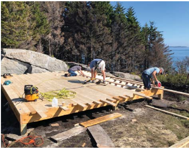
Completing the deck for the new shop
