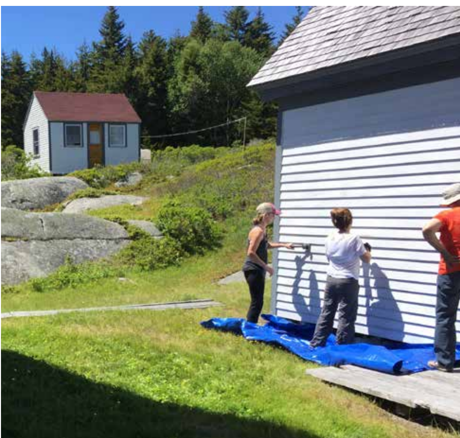
Volunteers painting. We try to paint one side of the Keeper's House every year.
