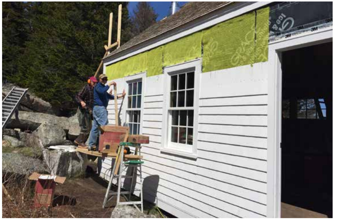
Volunteers work on shingling Yoder House II, the new workshop
