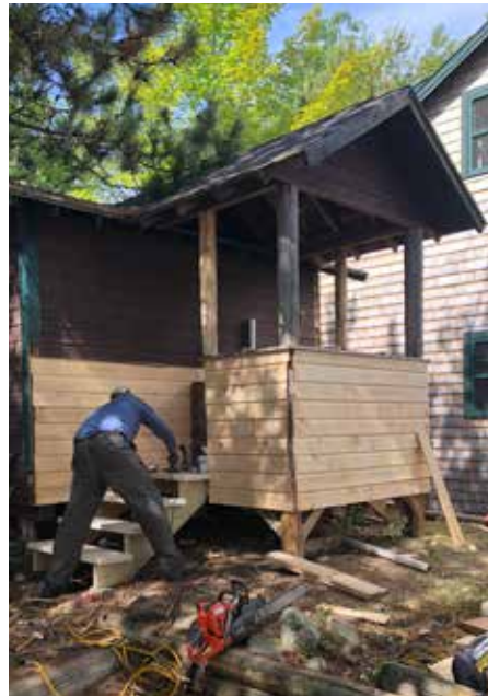
John Alsop building steps to the newly renovated Pump House
