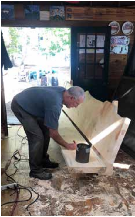
John Alsop at work on the new kitchen dock bench
