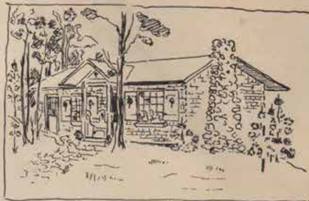
The Memorial Building
