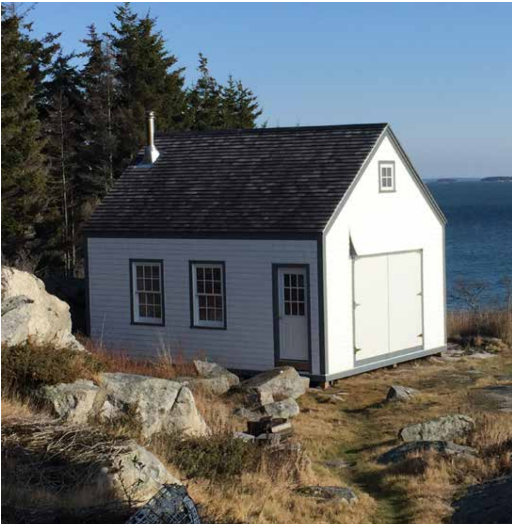
Yoder House II finished and ready for use as the workshop
