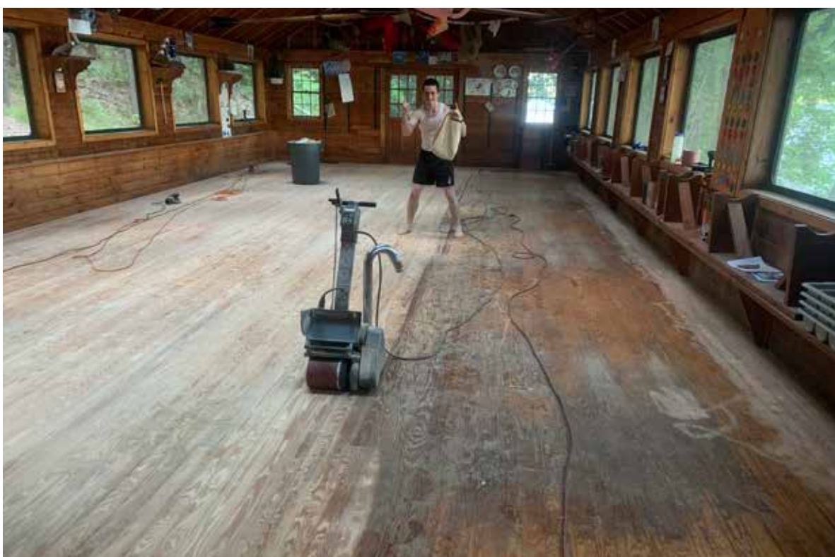
Projects head Miles Frank on the partially sanded Dining Hall floor
