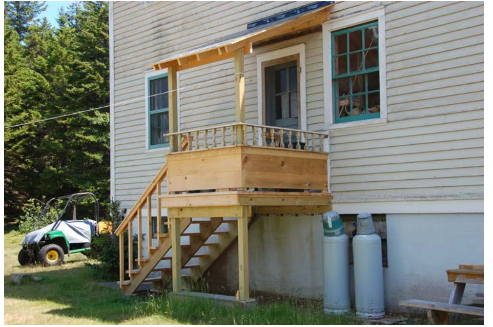
The new back porch and steps on the Barracks
