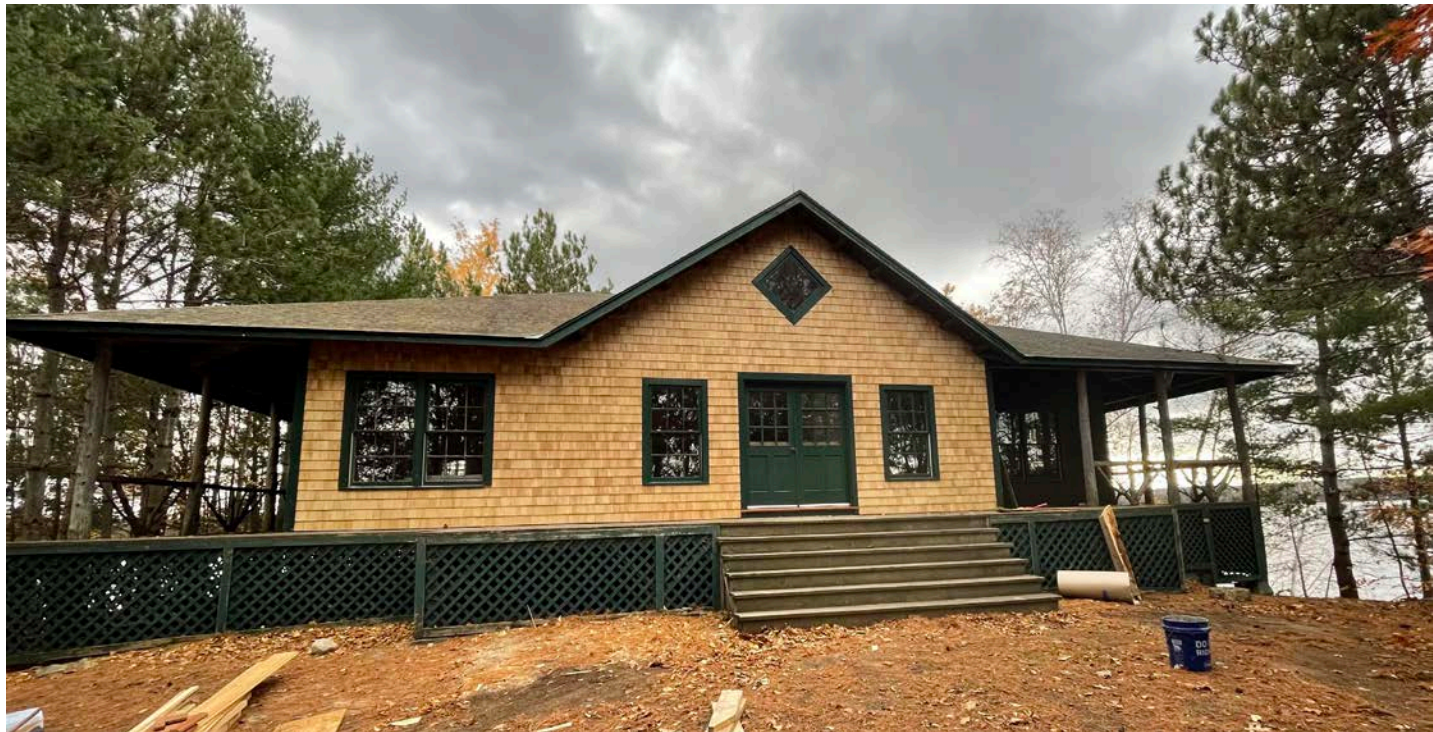
The newly shingled north side of Honk Hall
