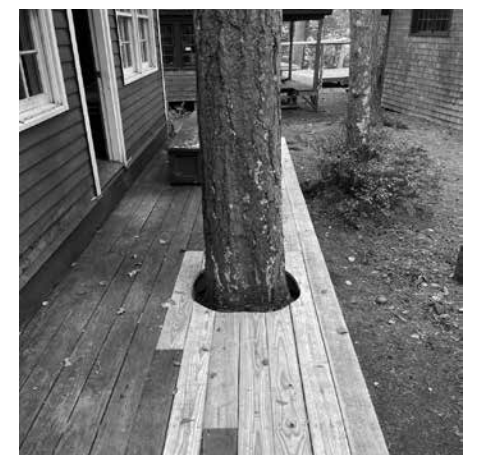
The Kopa Kababa porch after some much-needed repairs
